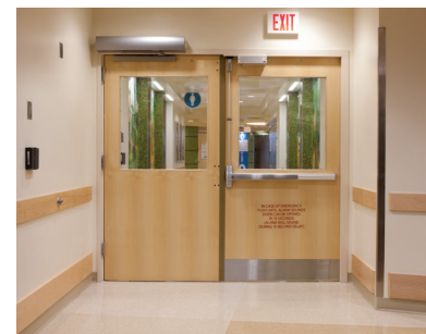
In the 2015 edition of the IBC, the activation time for delayed egress locks was changed from 1 second to 3 seconds, which is consistent with NFPA 101.
