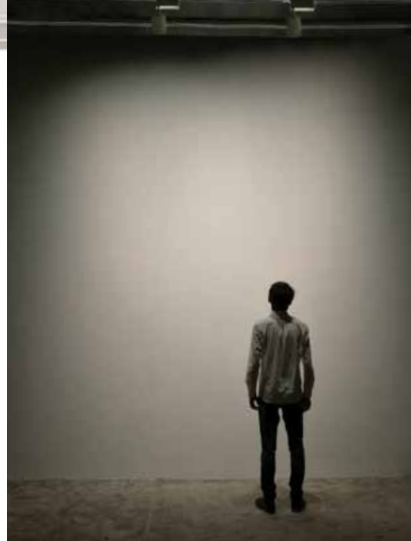
12ft wall illuminated with two WTK-6022A fixtures spaced 3 feet apart and 3 feet away from wall
